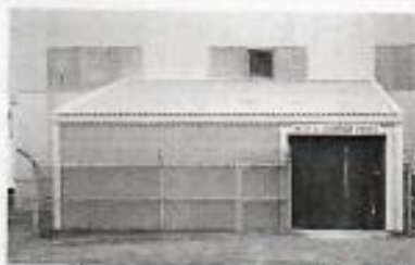
Above: the new grounds maintenance shed on June 13.
